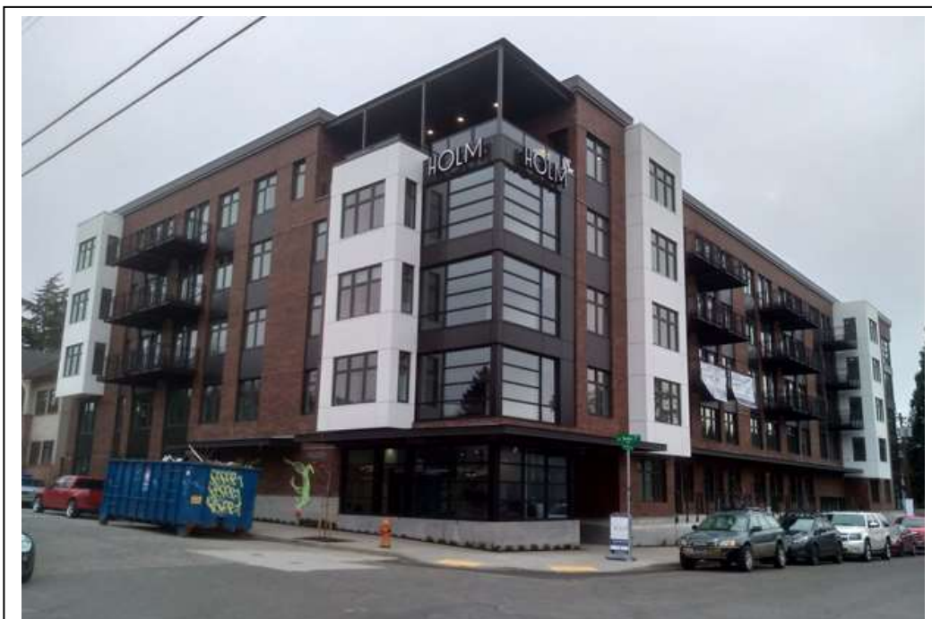
The FINISHED project!
