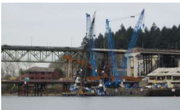
View of the east side construction from Powers Marine Park
