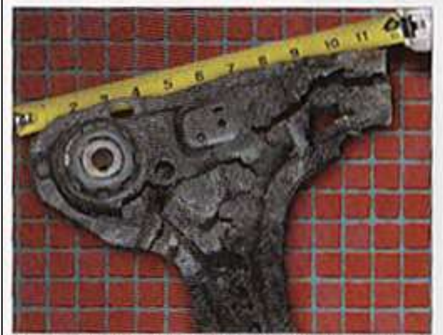
It can be tricky to see (and photograph) how extensively rotted a frame may be in a particular instance in the installed position. This corner of the subframe is designed not only to support the engine, lower control arm and steering rack, but also to absorb and redirect energy in the event of a crash. Don't send a customer back out on the road with a condition like this without a well-written waiver of liability. Better yet, don't send him back out like this at all.
