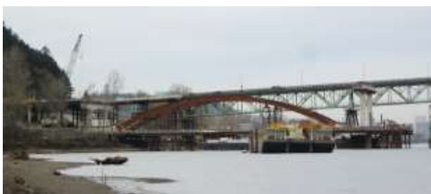
View of the east side construction from Powers Marine Park
