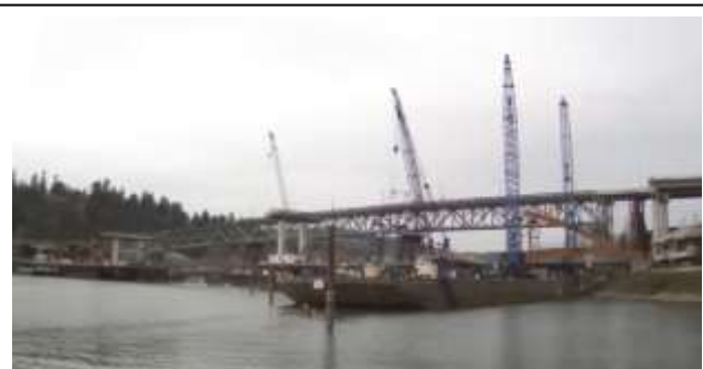
View of the east side construction from Riverpark Condos
