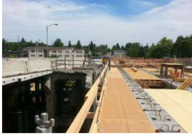
View looking west from the tip of the east side construction. You can see the old bridge and new bridge just inches apart. This small part of the old bridge will be one of the last remaining parts to be addressed, as described below.
