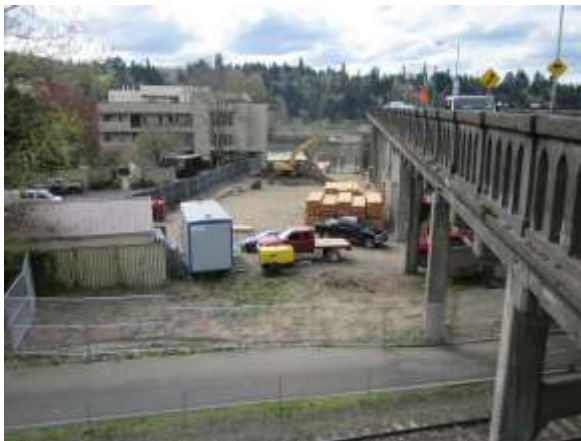
Construction staging on the southeast bank of the bridge
