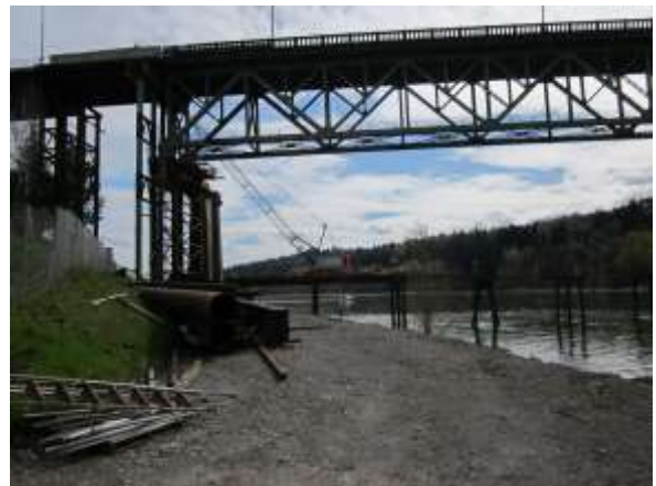
View of construction platforms from the northeast bank
