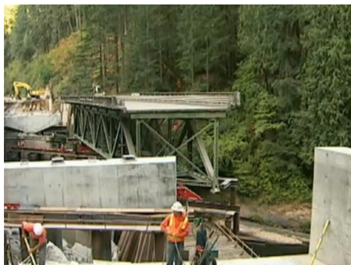
Elkton Tunnel West End Bridge Replacement
